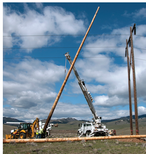
Crews for NorthWestern Energy replace poles on the Milltown-Idaho 161-kV transmission line. Photo courtesy of Susan Malee, NorthWestern Energy
