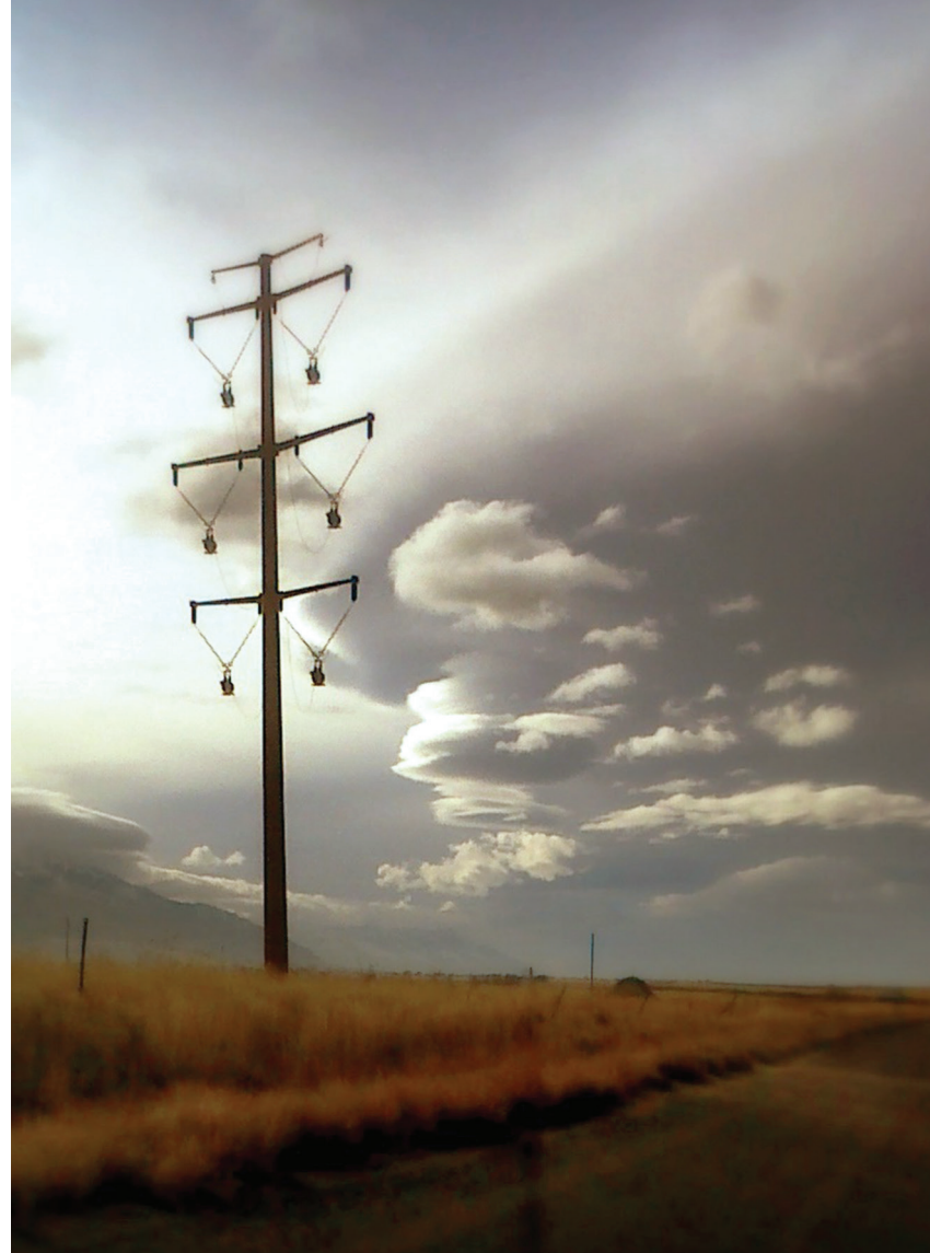
A 345-kV double-circuit mono pole steel structure with travelers in place awaits conductor installation on the Populus-Terminal 345-kV line in Utah. Photo courtesy of PacifiCorp
