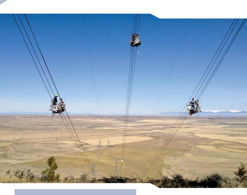
Above: Crews perform liveline spacer replacement on a 500-kV transmission line between switchyards in central Montana. On the cover: A segment of the 500-kV Mona-Oquirrh transmission line runs through Tooele County, Utah.
